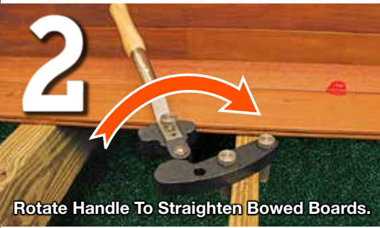
Position The HARDWOOD WRENCH™ On The Joist.
